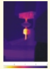
Thermal Image of Hot Spot
